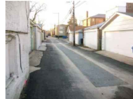
Permeable Concrete Center Trench in Concrete or Asphalt Alley
