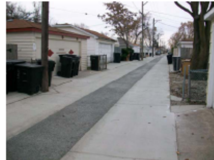
Permeable Concrete Center Trench in Concrete or Asphalt Alley
